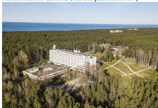
Figure 3-16 Building of the Jaunķemeri Rehabilitation Centre. Source: jaunķemeri.lv,
